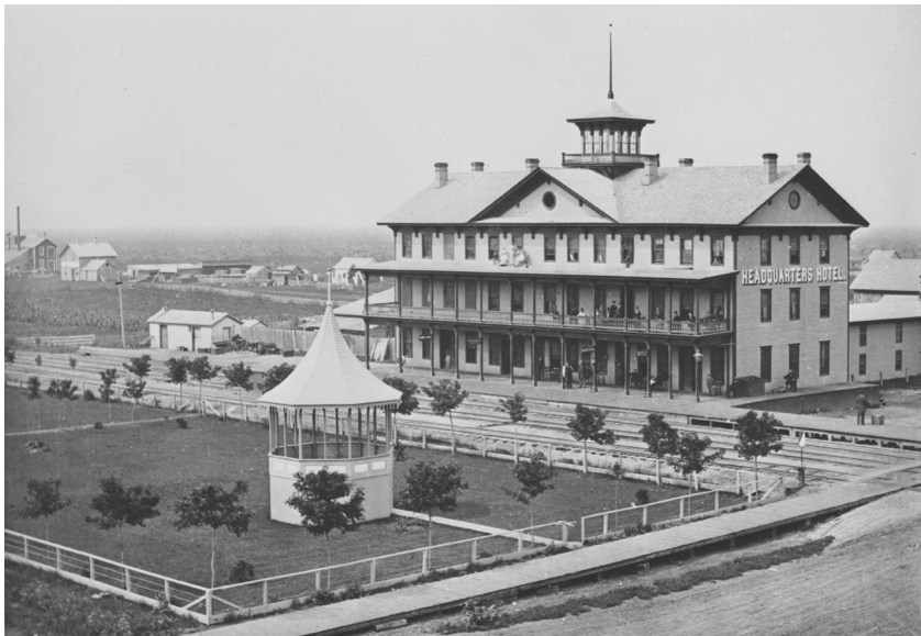
Headquarters Hotel and Northern Pacific Depot (1879) at the northwest corner of Broadway and Front Street (present-day Main). Photo courtesy of NDSU Archives.
